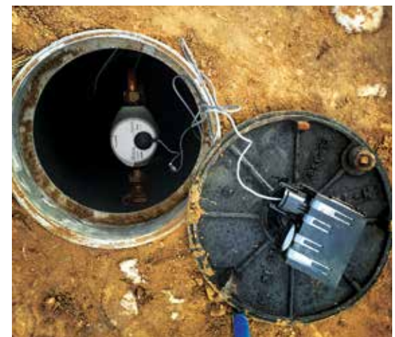
The smart water system installed in Evans allowed the utility to decrease estimated meter reads to 74 from 1,500.
